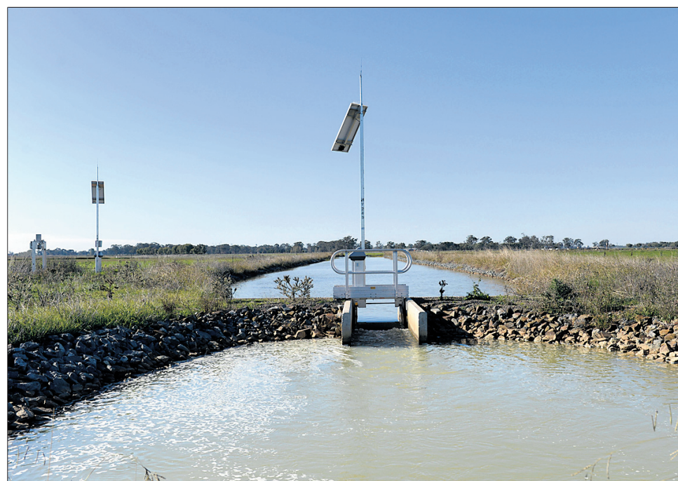
Four wheels were replaced with one automated gate.
